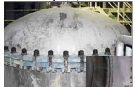
WEICON HB 300 - Repair of a vertical screen in a paper factory
