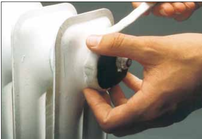
Sealing of a radiator leakage
