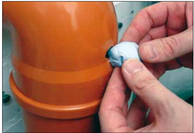
Repair of a PVC pipe
