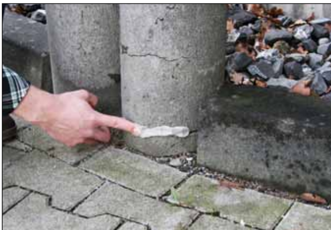
Sealing of a crack in concrete
